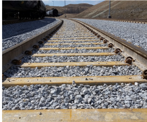
Completed steel tie track
