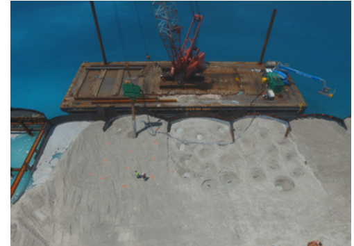
Figure 3. Typical view on vibrocompaction operation showing compacted cells
