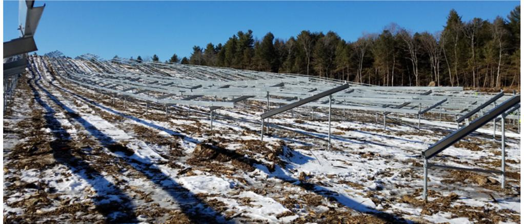
*Ground mount rack system supported on screw pile foundation*
