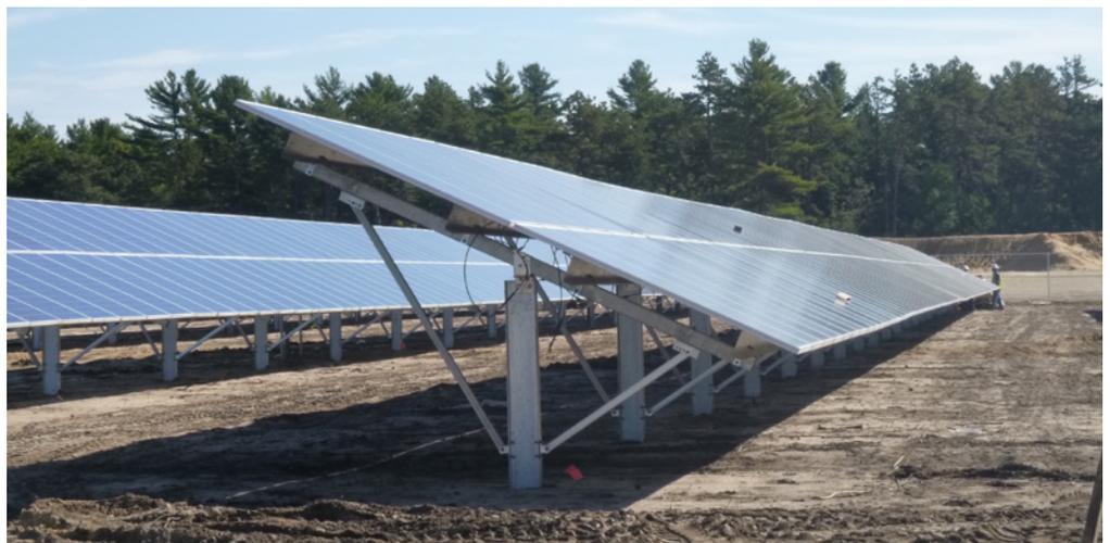
*Ground mount racking system and solar module supported on driven H pile foundation*
