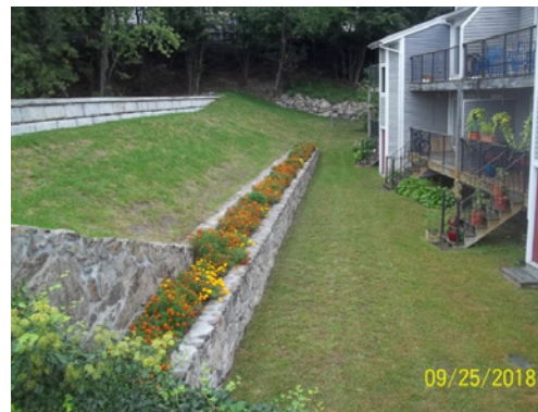
Left downstream embankment following removal of the upper portion of the masonry wall and regrading of the slope up to the top of the dam
