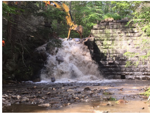
Controlled removal of existing masonry spillway.
