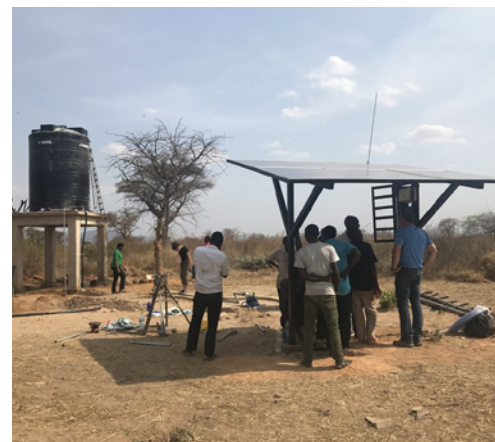
Installed storage tank and solar panels
