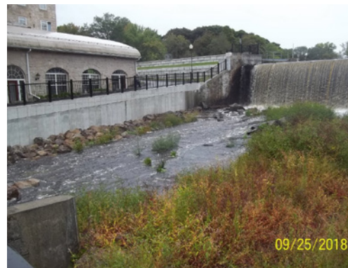
Reconstructed right discharge channel wall addressed collapsed segments of the wall.
