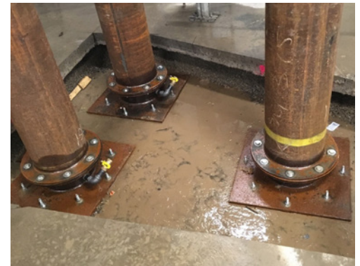
Standpipes enclosing the installed micropiles were anchored to the existing slab system.
