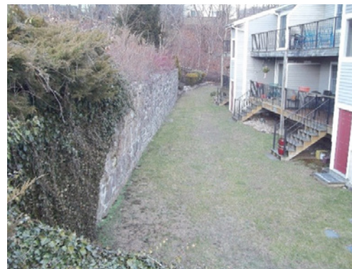
The left downstream embankment prior to repairs was found to have an inadequate stability factor of safety.
