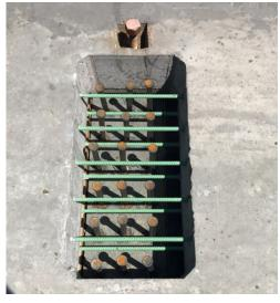
Shear studs installed on the existing beams at blockout of the precast deck panels.
