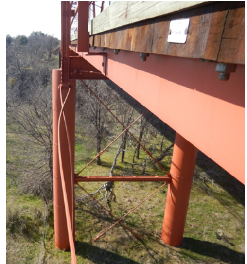
Figure 2: Lower chord eyebars designed to be in tension are bowed, and appear to be in compression.
