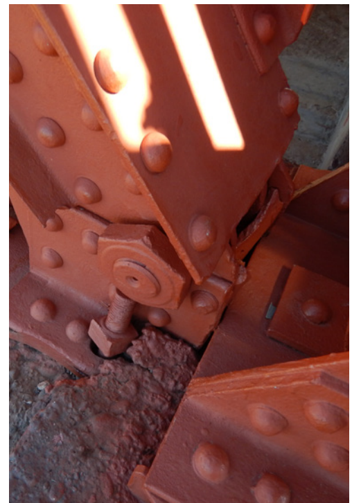
Figure 5: Expansion bearing from one span in contact with fixed bearing from adjacent span.
