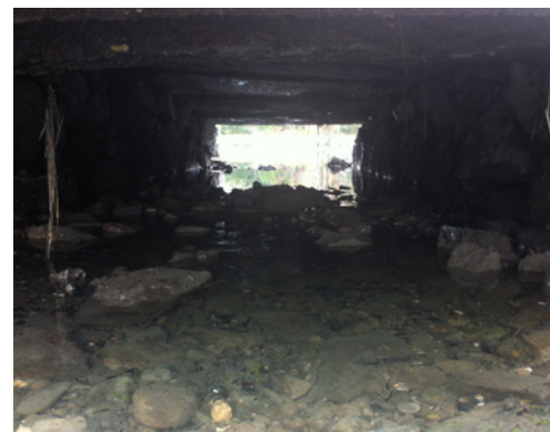
Old Shallow Granite Block Culvert
