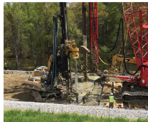
Figure 2: DMM Soil-Cement Wall Installation
