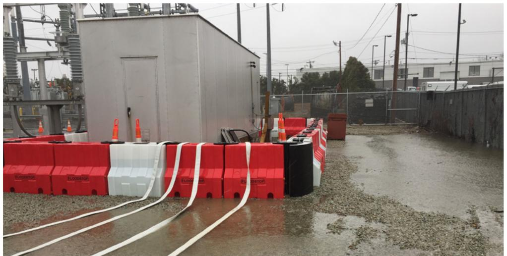
Water levels rising around Floodstop® barriers protecting critical energized equipment in Boston Harbor during Nor'easter Riley in March 2018
