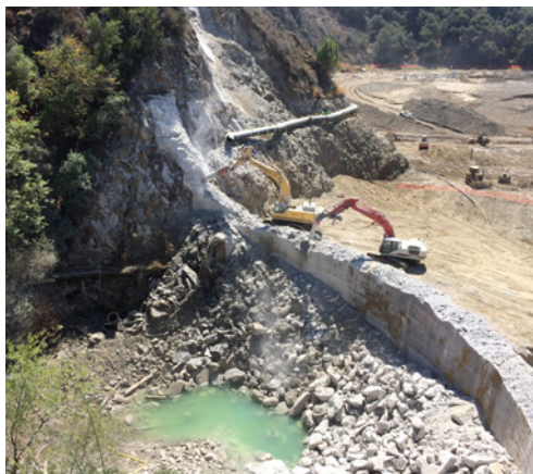
Figure 1: Removal of the dam structure.
