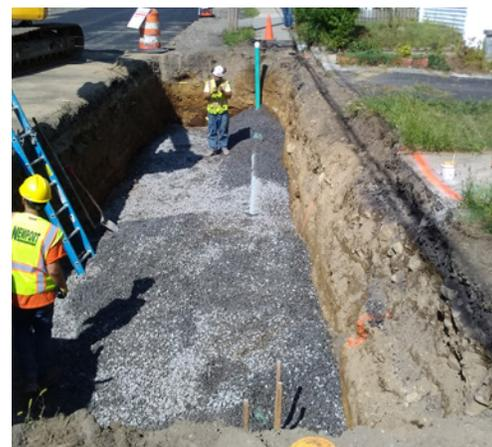
Tree trench underlain by gravel to enhance subsurface storage and increase rate of infiltration (photo courtesy of Horsley Witten Group)
