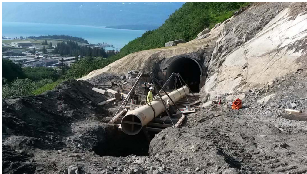
Penstock installation outside of the tunnel along the upper access road.
