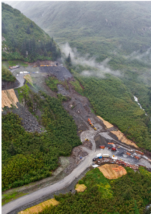
Aerial view of lower half of Allison Creek Project; lower right: power house & access road; upper left: lower tunnel portal.
