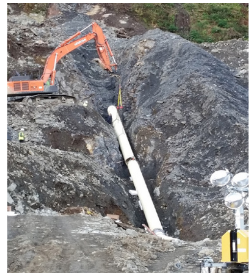
Portions of the Penstock were trench buried on steep slopes such as this 60% grade; others traveled through the underground access tunnel.
