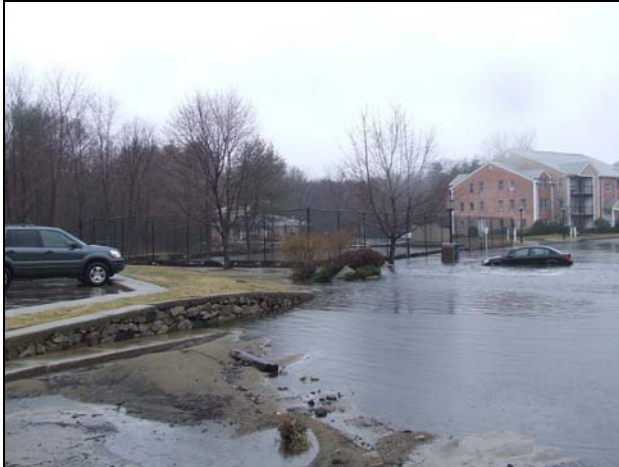
Car trapped in the wake of failed Canton dam Photo Credit Robert S. Stephens, PE
